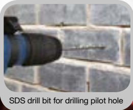
SDS drill bit for drilling pilot hole
