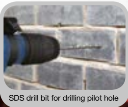
SDS drill bit for drilling pilot hole
