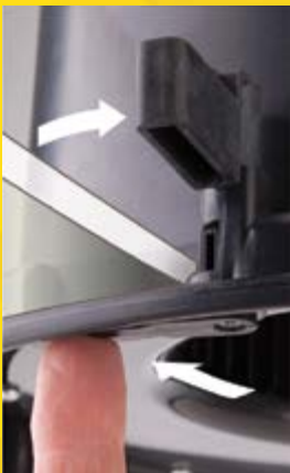
Rotate swing clips to hold fan body in place.
