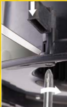
Tighten screws so clips clamp onto ceiling board.
