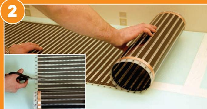
2 Unroll the **ECOFILM<sup>PRO</sup>** and cut to required lengths. Cover the floor area with elements laid in parallel. Elements should NEVER overlap.
