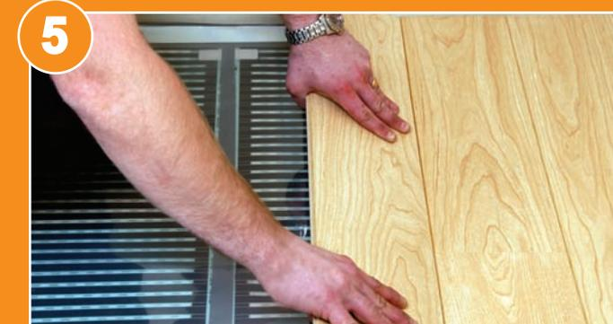
5 Lay the floor covering as soon as possible to prevent damage to the element.
