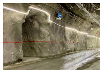
HALO Underground Mining
