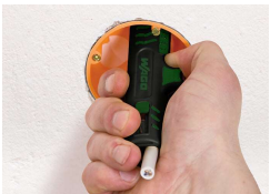
Stripping a cable sheath.
