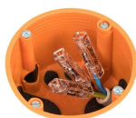
Extending short wires.
